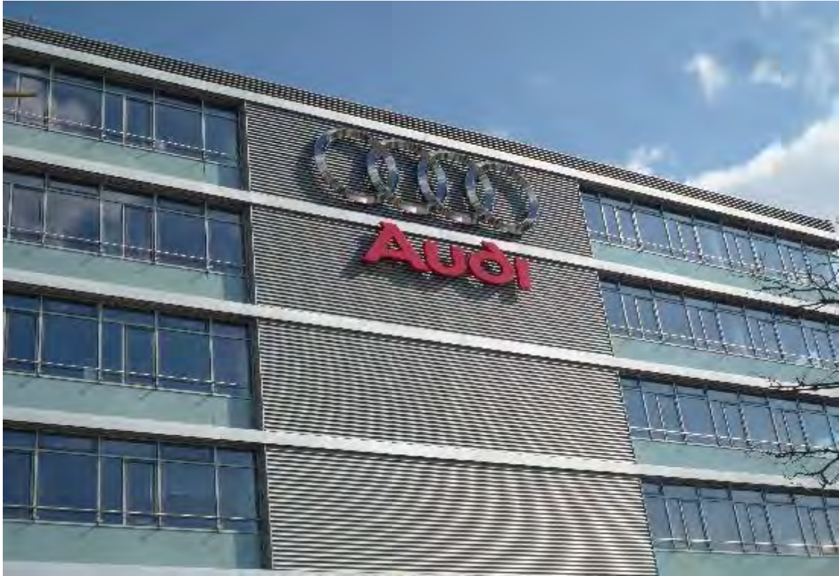
Headquarter of Audi in Ingolstadt (Germany)
